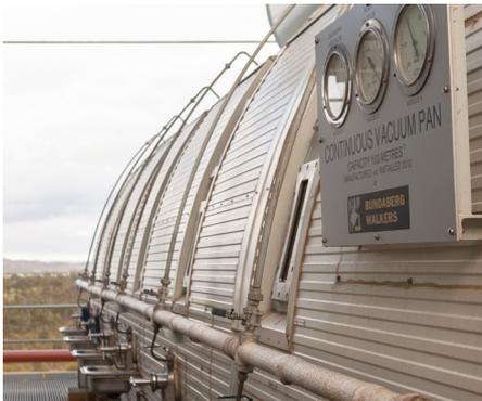
**Sugar Research Institute's Continuous Vacuum Pan design produces high massecuite exhaustion, consistent crystal size and improves energy efficiency.**
